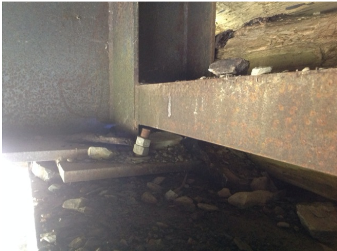
left bank upstream bearing bolts
