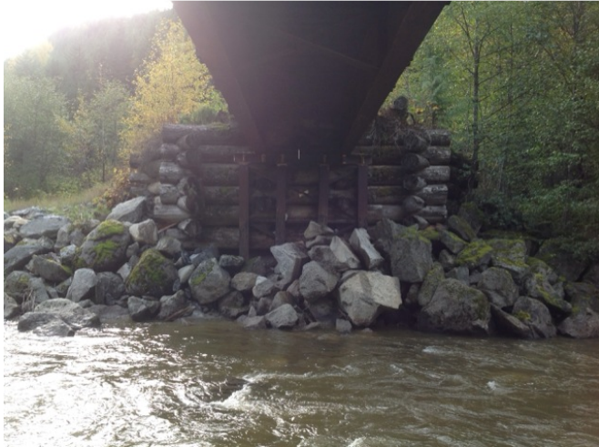
Left Bank Abutment when facing downstream
