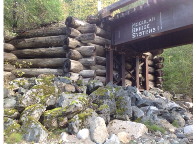
Right Bank Abutment when facing downstream
