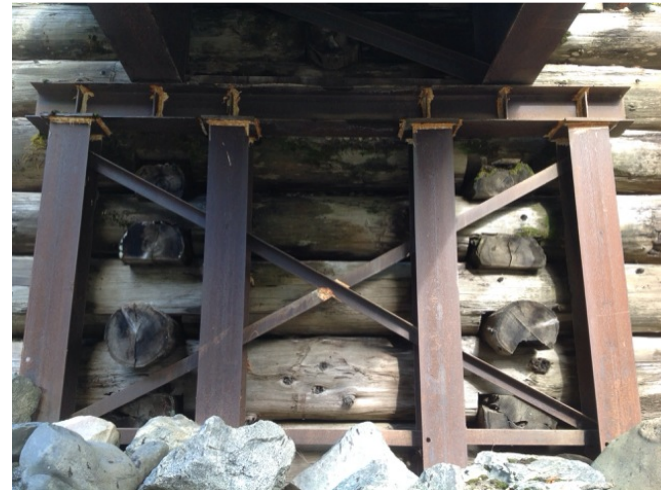
Right Bank Abutment when facing downstream
