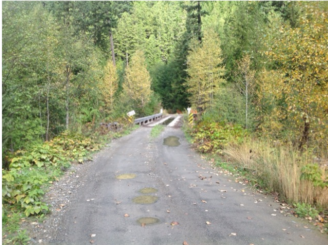
Approach from Left Bank when facing downstream
